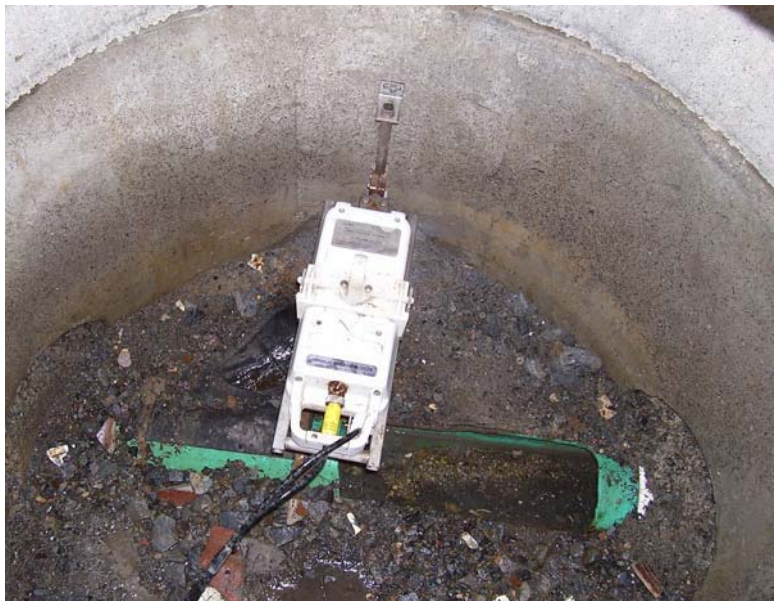
Heavily debris-laden flow in Whitehall, NY monitored by non-contact Flo-Dar sensor utilized in DDS program.
