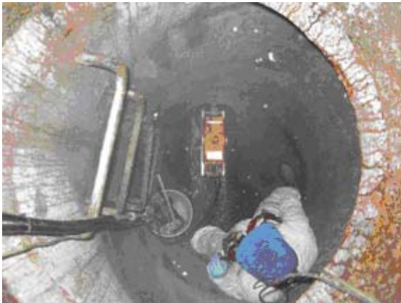
DDS Meter Install Hilliard Ohio (Intersection Scioto & Darby Creek Rd)
