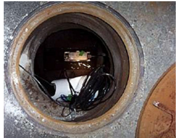
Hach Data Delivery Services provide a maintenance-free Flo-Dar flowmeter plus 24/7 web-based access to data.
